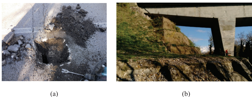
Fig. 11. Details of the gap between the deck and the hillsides.
