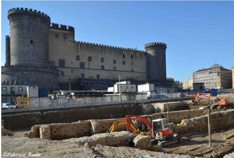
©Fabrizio Reale Fig. 10 – Aerial view of excavation
