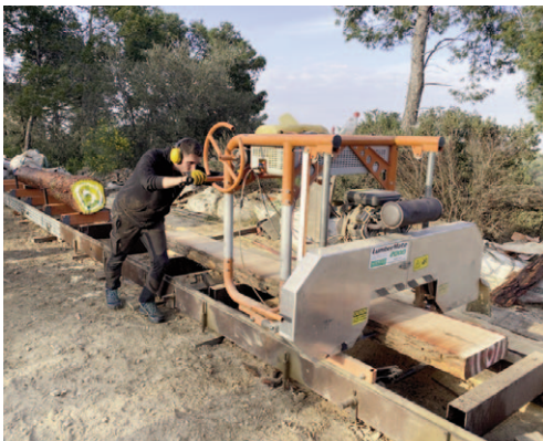
Fig. 4 | VQC: In situ tree trunk cutting process for construction components (credit: A. Goula, 2020).
