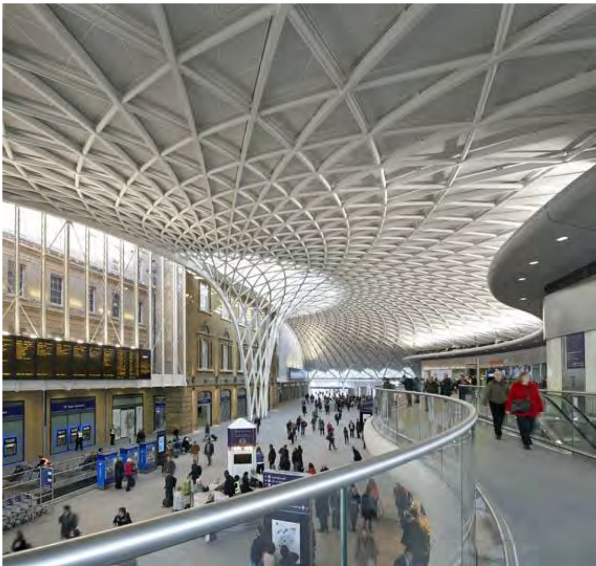
Londra, Kings Cross Station
