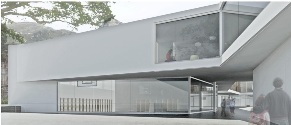
Figure 3. The Entrance to the New School
