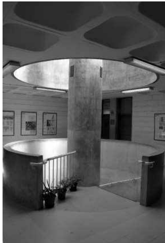
José Gomes Ferreira School interior stairs
