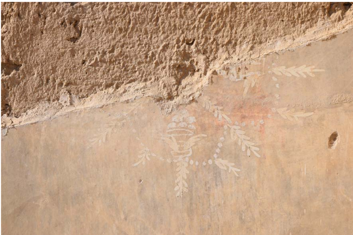
Fig. 27 - Room AU12Nα, West wall, detail
