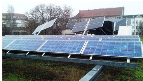
Fig. 2 - Ufa Fabrik, Green roof and fixed and mobile PV panel system (Photo F. Dell'Acqua, 2018)
