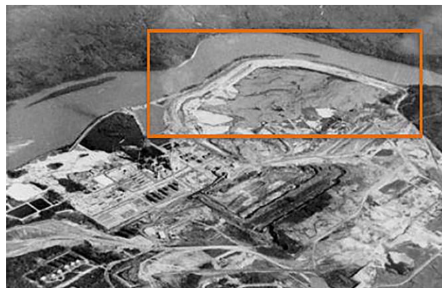
Figure 2. Aerial view of Tar Island Dyke in the early years (McRoberts et al. , 2017)
