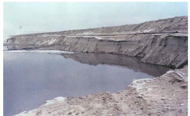
Figure 8. Example of steep as-constructed cell slope with pond at toe (photograph courtesy Ed McRoberts)
