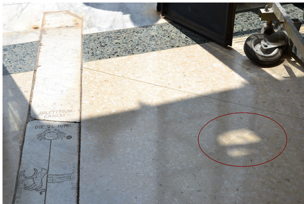
Fig. 7 The inaccurate luminous Sun's image that today appears on the floor (some minutes before noon), in consequence of the erroneous attempt to restore the original functionality of the meridian line. Photo: Alessandra Pagliano
