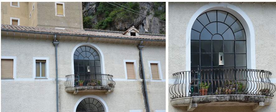
Fig. 20 Photomontage of the diverter object on the transparent surface of the window of the Abbey of Cava de' Tirreni. Image: Angelo Triggianese
