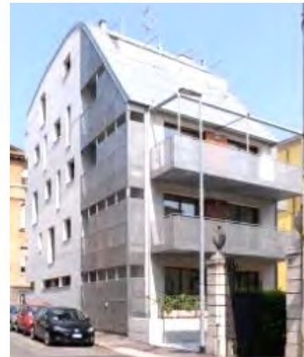
Fig. 122 Edificio residenziale e terziario in calcestruzzo a faccia vista a Bergamo (classe A) / Residential and tertiary building made by concrete to face situated in Bergamo
