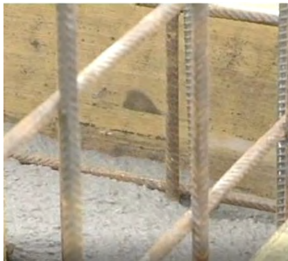
Fig. 7, 8 e 9 Proprietà reologiche del calcestruzzo autocompattante / Self compacting concrete rheological properties a) filling ability; b) passing ability; c) stability
