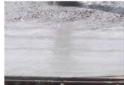
Fig. 6 Scorrimento del calcestruzzo autocompattante / Self compacting concrete sliding
