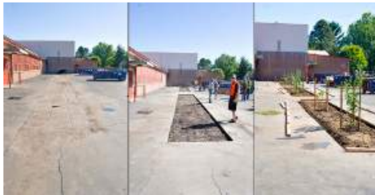
Fig. 81: Depave process example (source: https://content.yardmap.org/learn/what-is-and-how-to-depave/ ).
