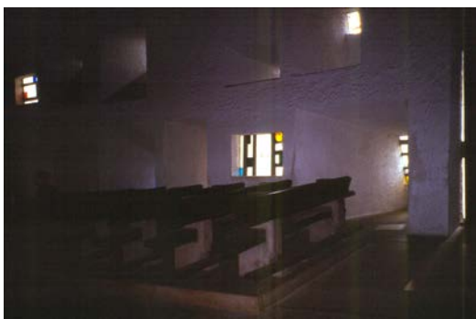
Fig. 2 - The white plaster on the inner surface of the Ronchamp Chapel.
