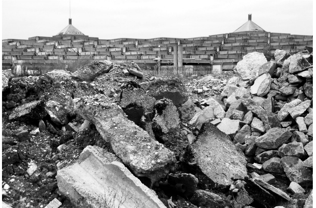
Fig. 2 - The Former Cattle Market of Padova, I (photo by S. Antoniadis, 2012).
