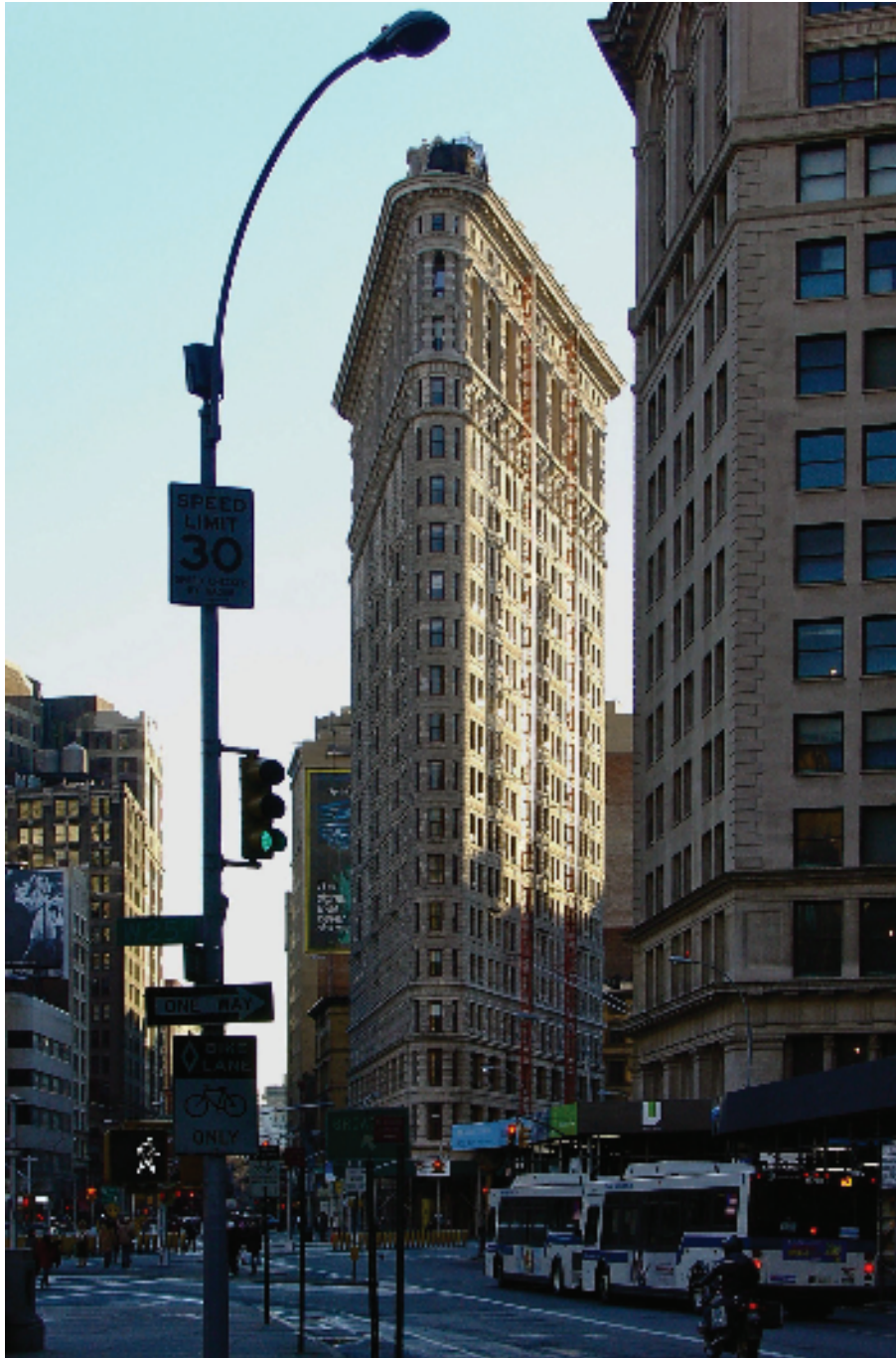
01_Flatiron Building, New York, 1902. foto Paolo Giardiello
