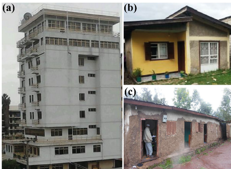
Fig. 9 Typical buildings in Addis Ababa identified as: a Condominium, b Villa, c Mud and Wood
