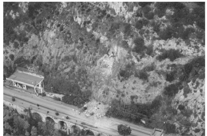
Figure 3. The rockfall occurred on 18 th February 2014.
