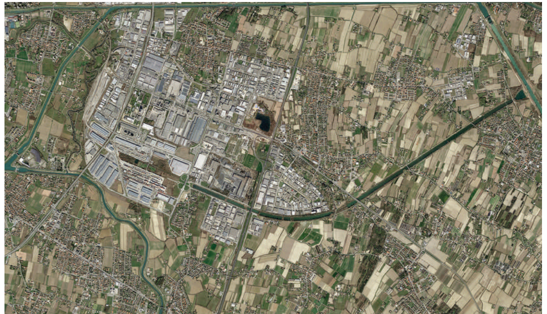
Fig. 1 - Western stretch of the Padua-Venice waterway, from the industrial district of Padua and Vigonovo (PD). Aerial view. (source: Google Earth, 2016).
