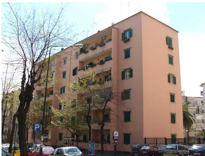
Fig. 6 One of the buildings of Rione Gemito
