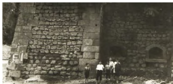
Fig. 5– De Luca, East front of Sant'Antonino bastion, 1920, detail (Fiorentino, 1991).
