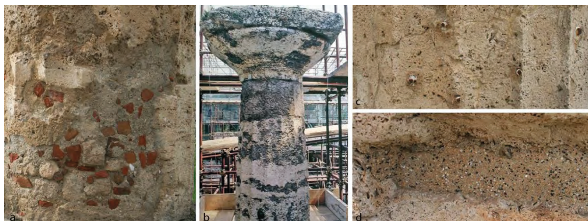
Figure 2: a) temple of Athena, column of the northern side. Addition in fragments of bricks and concrete (1926); b) temple of Neptune, column of the upper order. Integrations in bricks and concrete (Fifties); c) temple of Athena, column of the eastern front. Reinforced perforations (1962); d) temple of Neptune, column of the northern front. Integration made of lime mortars (1997-2002).
