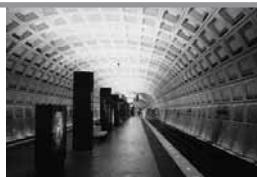
1976_harry weese & associates_ metrorail system_washington
