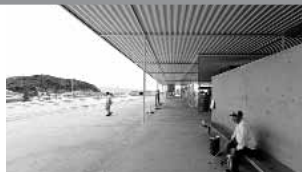
2004_SANAA_ferry terminal_ naoshima
