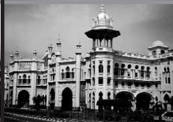
1910_a.b. hubback_kuala lampur railway station_malaysia
