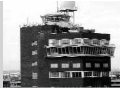
1955_f. gibbero_heathrow control tower_londra
