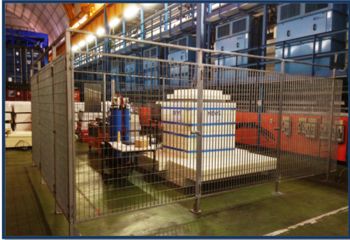
Figure 3. Picture of the shielded structure installed in the underground Hall B at Gran Sasso.
