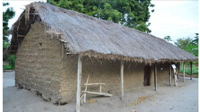
Figure 2. A Kwere e Doe-Bantu house - Nyumba Ya Wakwere Wadee. Communities resides in Coastal Regions of Bagamoyo and Kibaha districts
