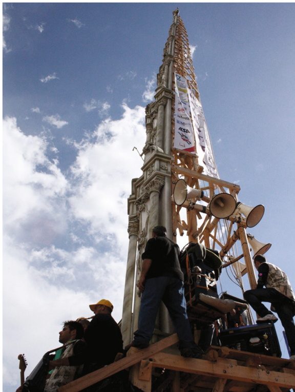
Fig. 1. (Left) A “Giglio” of Barra machine: on the right the wooden skeleton, on the left coloured coating of papier-mâché, covering only the front of the machine.
