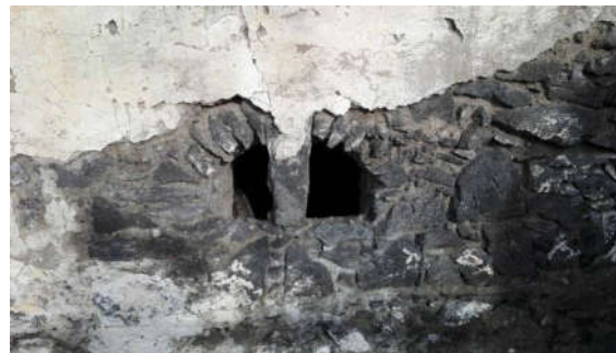
Fig. 16 Opening with lowered arch / Apertura con arco a sesto ribassato
