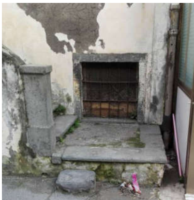
Fig. 15 Opening with wooden architrave / Apertura con architrave in legno
