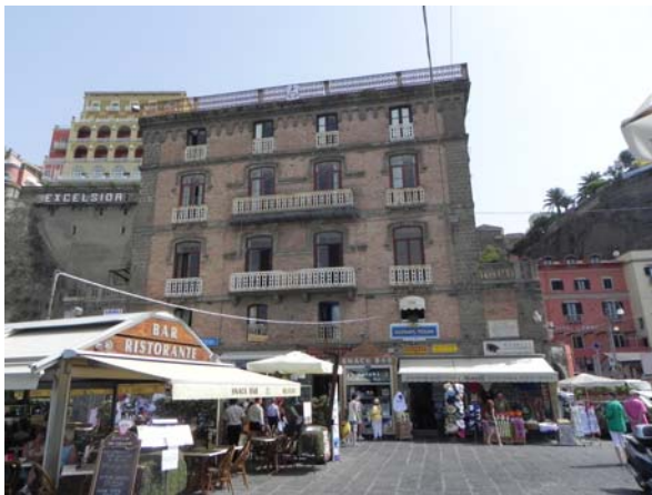
Fig. 1 – Marina Piccola Port area.
