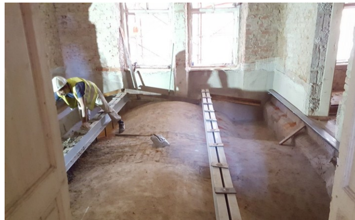
Fig.12 Reinforcement of the vault extrados
