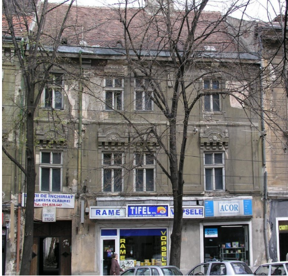
Fig.1 Front view of the 1 st studied buildings
