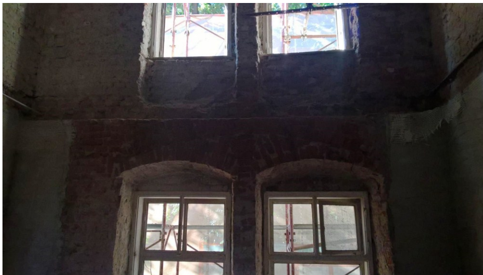
Fig.5 Consolidation of the ground floor corners
