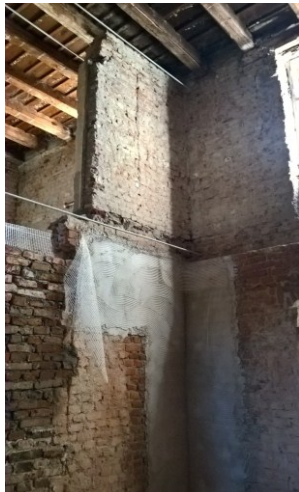
Fig.6 Consolidation of the corners
