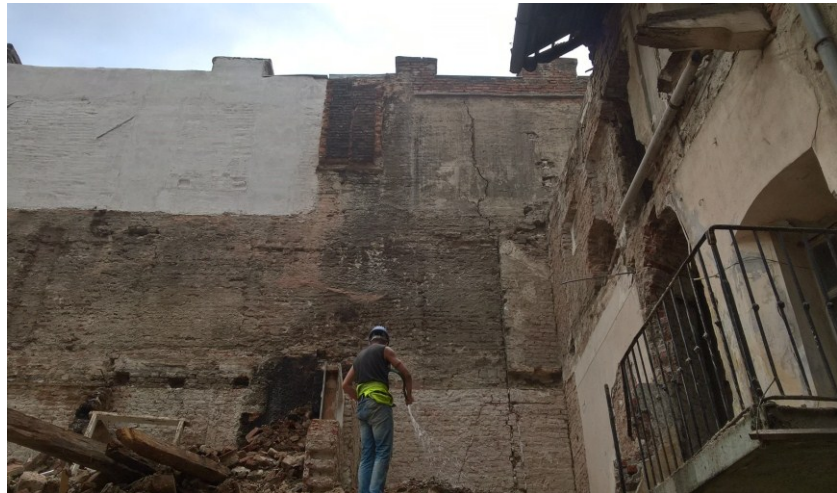
Fig.7 Consolidation of the exterior walls
