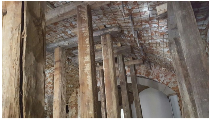
Fig.11 Reinforcement of the vault intrados
