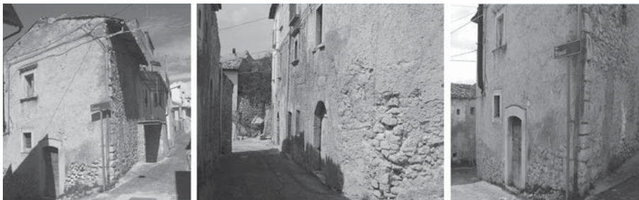
Fig. 9 Main views of the aggregate type B
