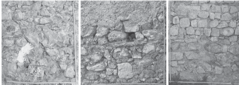
Fig. 7 Typical masonry textures
