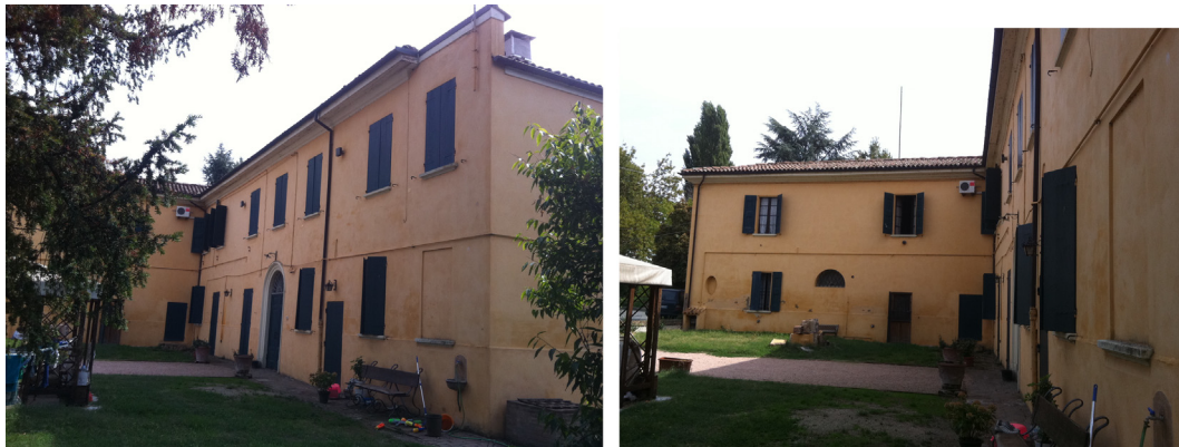
Fig. 2. Views of the building facades related to its residential part.
