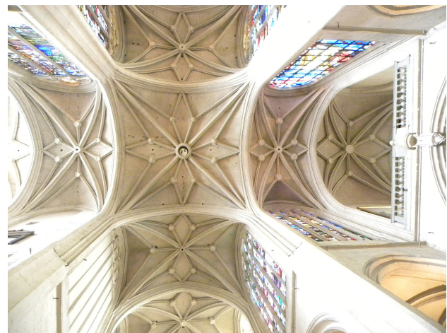
Figure 4 Paris St. Gervais et St Protais transept's rib vault system.
