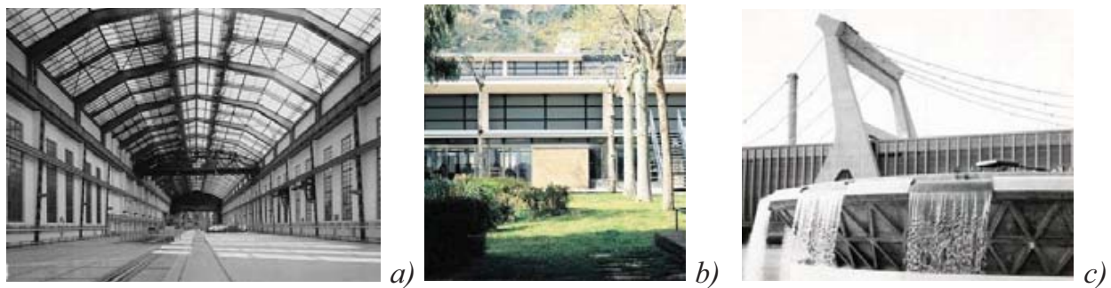
Fig. (2). The AEG turbine factory in Berlin (1909) [5] (a); The Olivetti factory in Pozzuoli (1951-1954) [6] (b); The Burgo paper mill in Mantova (1961) [7] (c).
