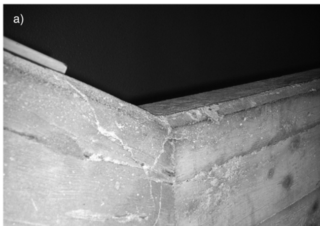
Fig. 6. Cracks in the staircase beam (a) and in a ground storey beam external to the school (b). Fessure in una trave delle scale (a) e in una trave a piano terra esterna all'edificio (b)
