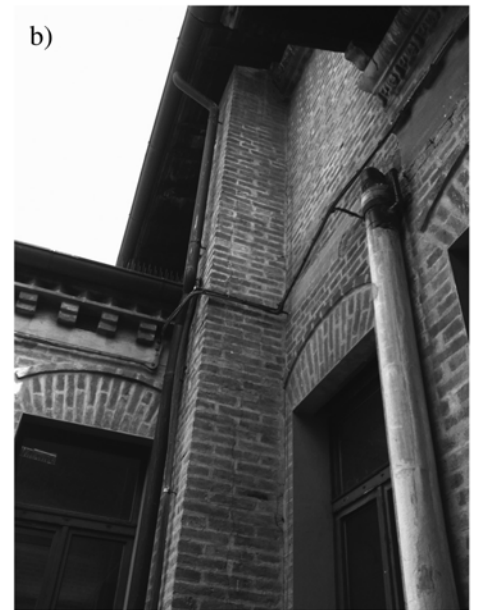
Fig. 21. A very large crack between two masonry walls (a) and a vertical crack between the chimney and the façade (b) of the primary school “Battisti”. Scuola elementare «Battisti»: una fessura molto larga tra due pareti in muratura (a) ed una fessura verticale tra canna fumaria e facciata (b).
