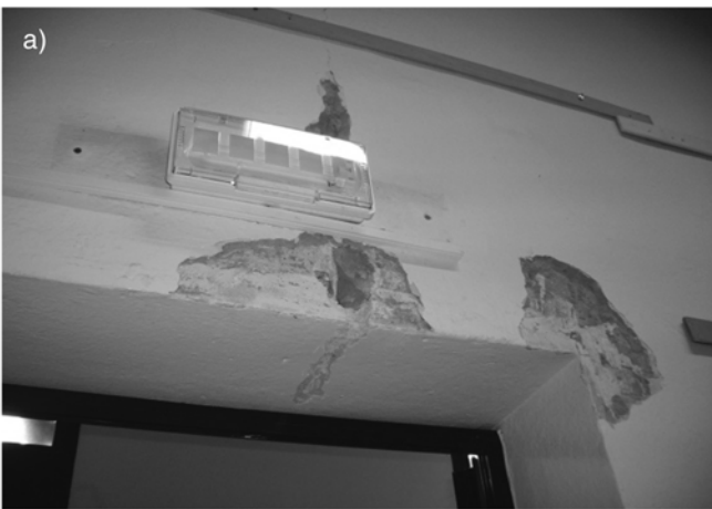
Fig. 10. Architrave (a) and wall-floor (b) cracks. Fessure in architravi (a) e tra pareti e solette (b).
