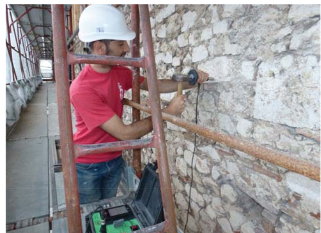
Figure 7. Example of sonic/ultrasonic test.
