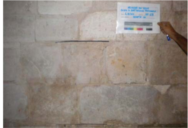
Figure 5. Sant'Eusanio church ( DS masonry).
