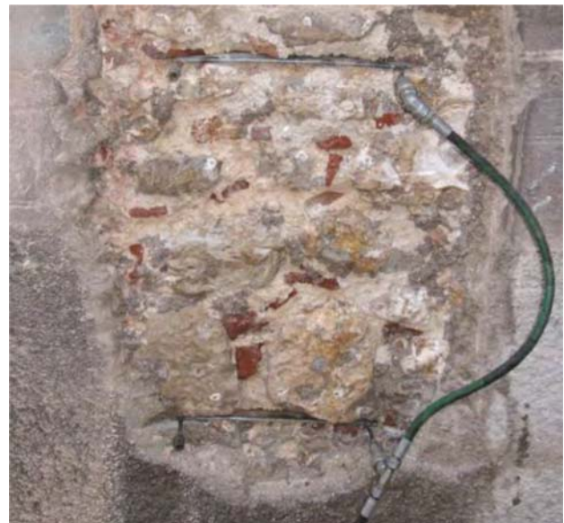
Figure 2. Santa Maria del Suffragio church ( T1 masonry).
