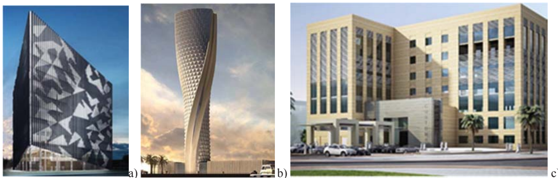
Figure 4. On-going NPP0064 project: (a) Mwani building, (b) Control tower, (c) Custom building
