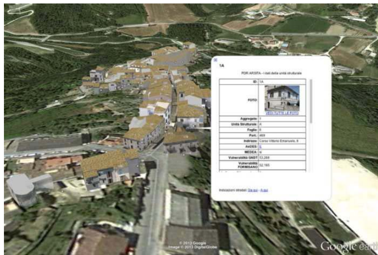
Figure 2 The 3D building inventory model of Arsita (see online version for colours)
