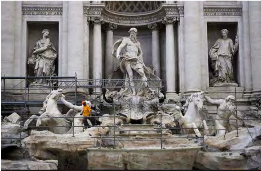
1. restauration works in Fontana di Trevi, 2013, source: tg24.sky.it
