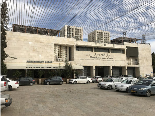
Figure 1. Photograph of the Peace Center overlooking "Manger Square", in the Bethlehem City Centre.
