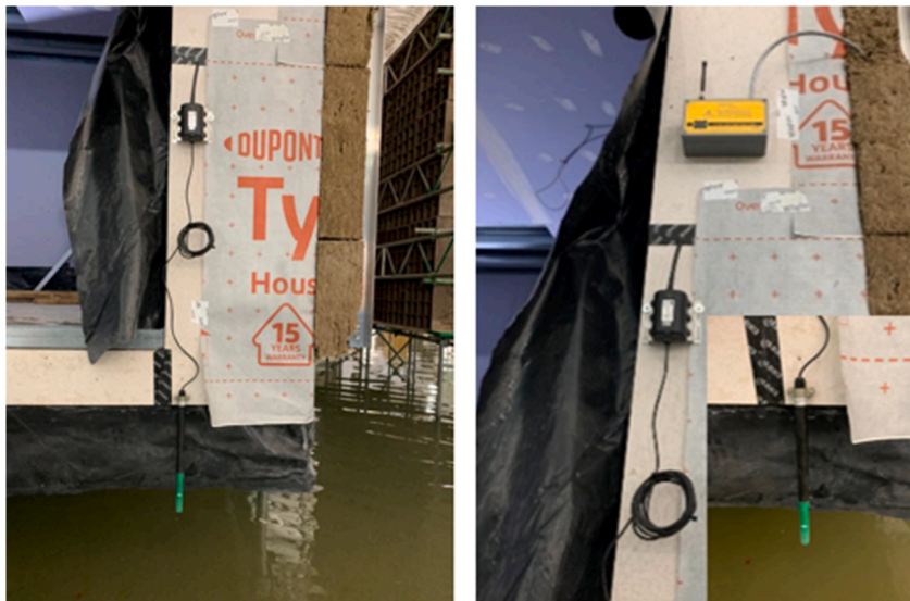
Fig. 8. Piezometer and its system positioned outside the FAP modular system.
