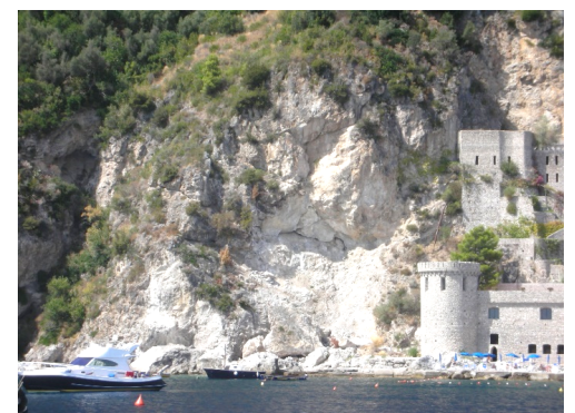
Fig.6 – Rockfalls affecting a coastal stretch in Conca dei Marini.
