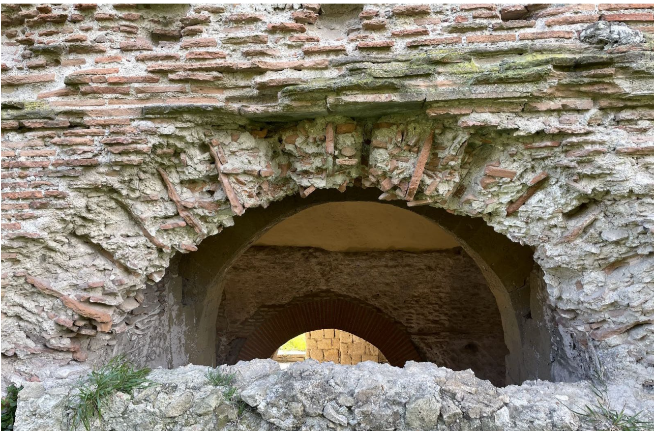
Figure 18. View of arches of the façade of the ambulacrum
