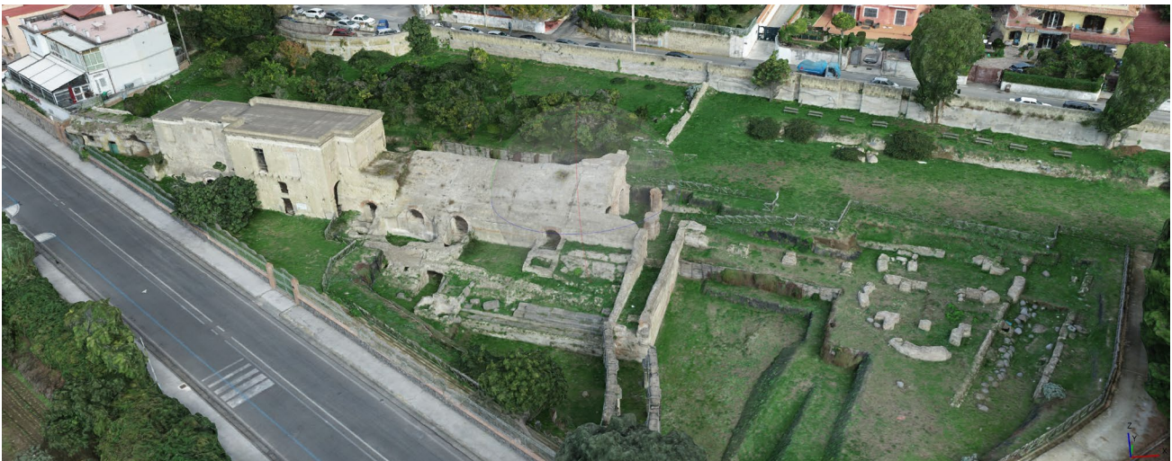
Figure 7. Perspective view of the dense point cloud from the RPAS (Remotely Pilot Aircraft System) of the Stadium of Antonino Pio.
