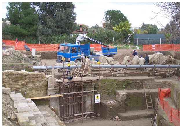
Figure 5. View of the reconstruction by anastylosis of one of the triumphal arches, 2007 (Archive of the Archaeological Superintendency of Naples)
