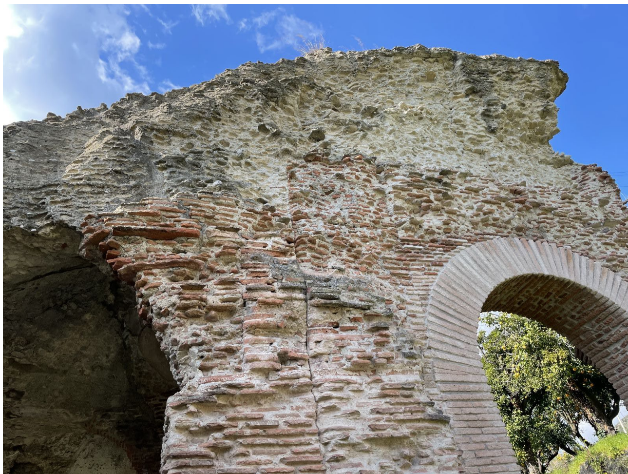
Figure 20. View of the outer wall of the ambulacro. Note that the two masonries are not joined
