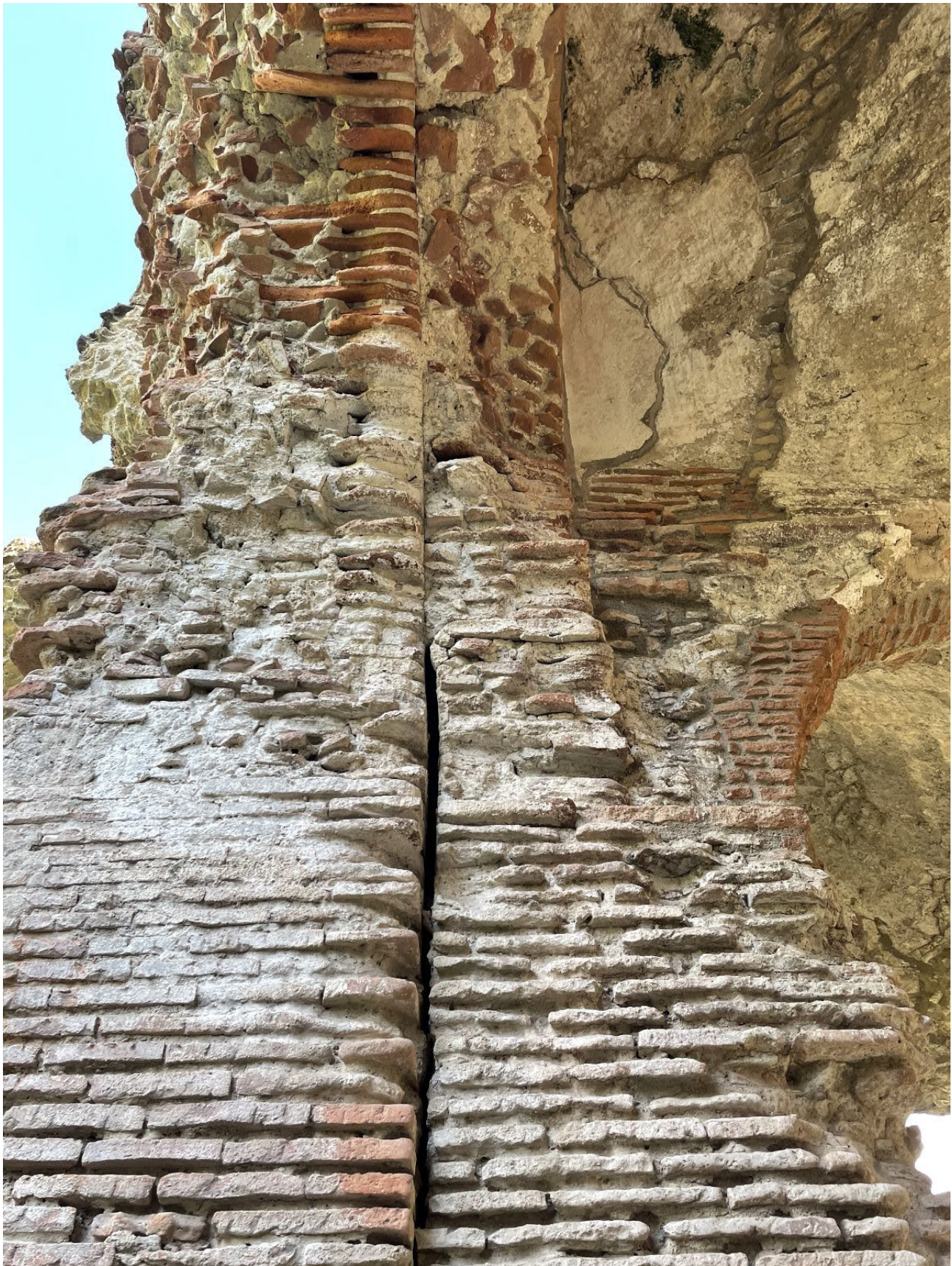
Figure 19. View of the inner side of the brickwork pier of the ambulatory arch. Note that the two masonries are not joined
