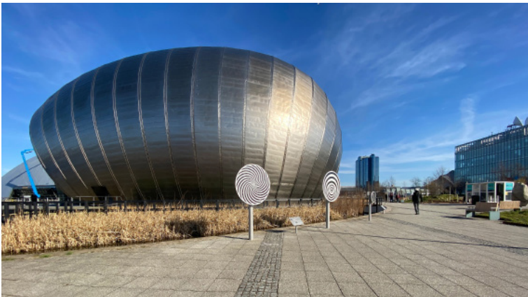
Fig. 3 Glasgow Science Centre. Outer Space (Source: Author).
