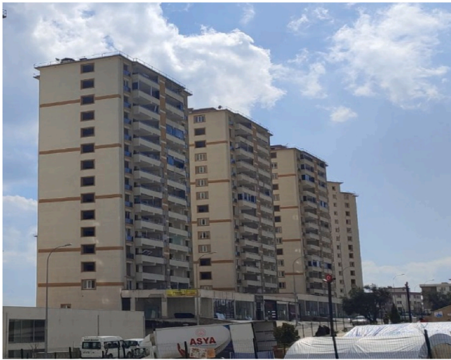
Fig. 1. Examples of cast-in-place tunnel-form buildings after experiencing strong earthquakes and aftershocks: Turkey, 2023.
