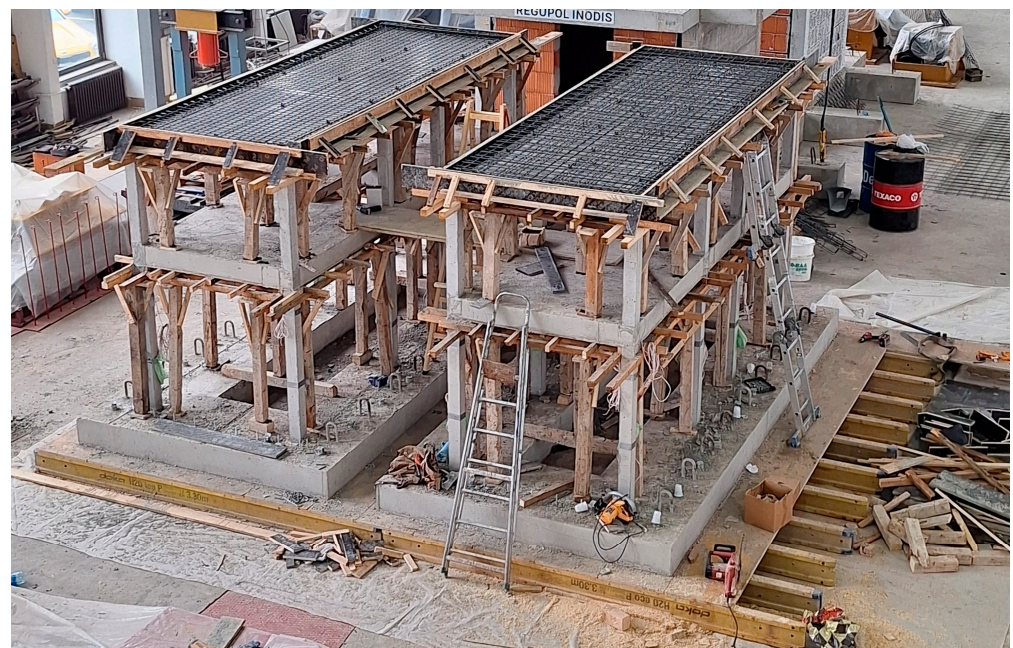
Figure 3. Building of the RC structure.
