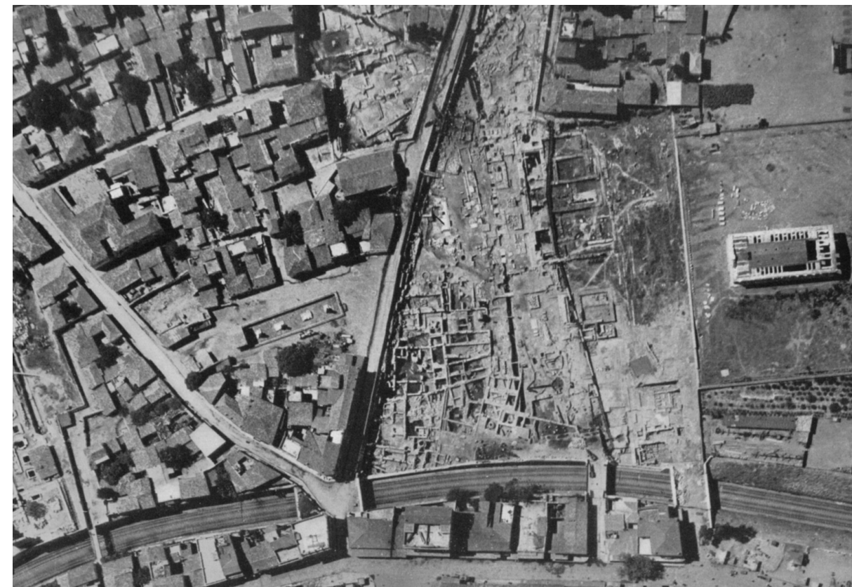
Figure 4. Initial demolitions in the northern area of the Agora excavations. From: Schear, 1933 (American School of Classical Studies at Athens: Agora Excavations).
