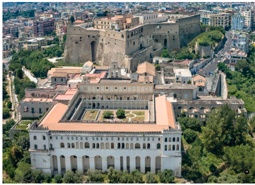
(a) A view of the San Martino Charterhouse exteriors.
