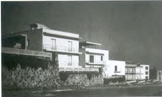
View from via Petrarca: the traditional party wall in Vesuvius stone and the experimental construction, late 1940s.
