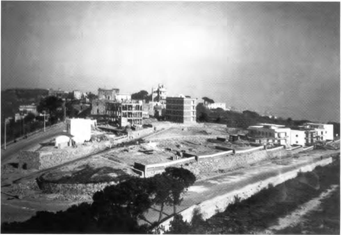
The experimental housing under construction, late 1940s.
