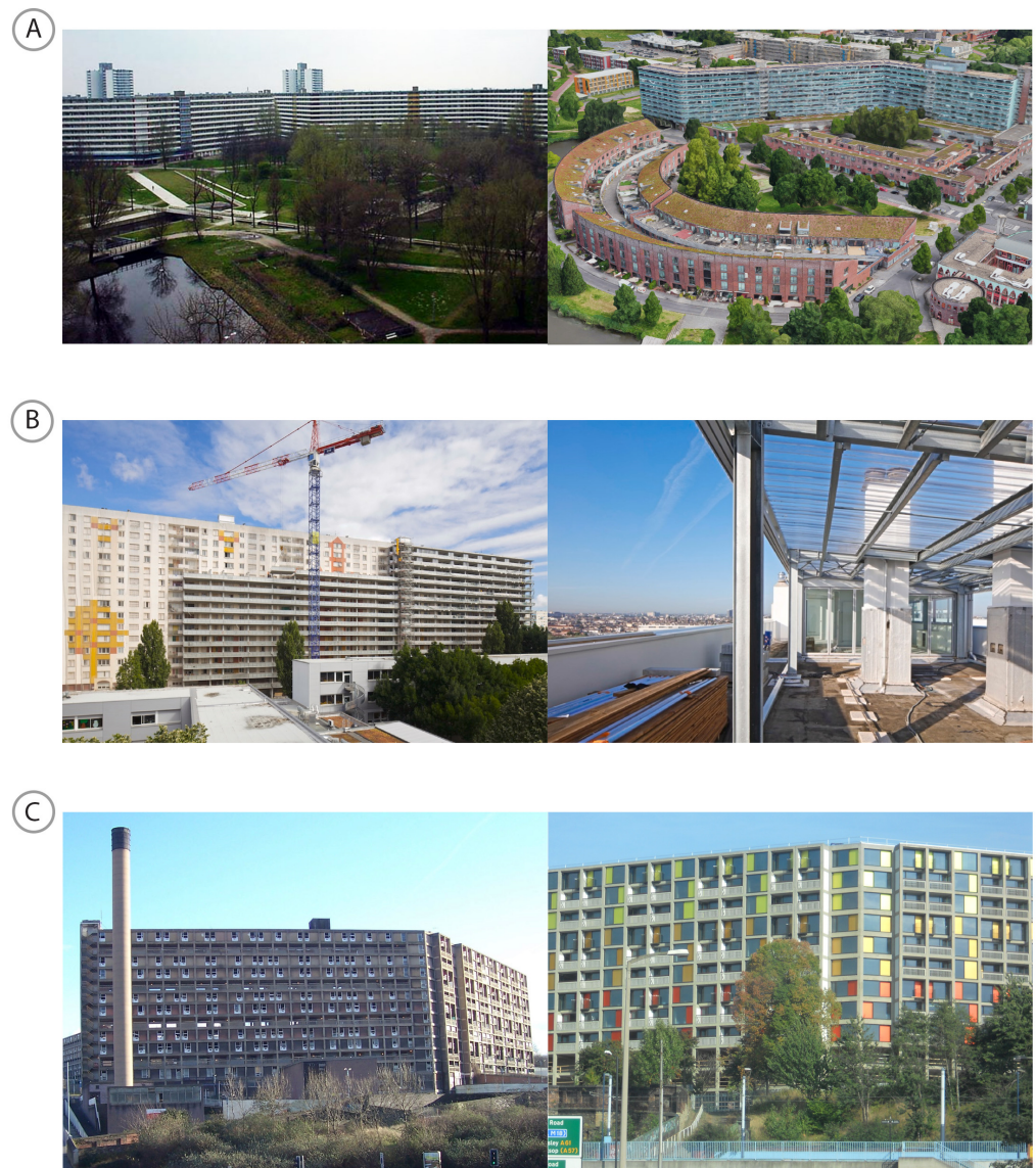
Figure 1. Some examples of best practices: (A) Bijlmermeer in Amsterdam (picture left taken from [29] and picture right taken from https://www.google.com/maps/ (accessed on 28 December 2023)); (B) Lacaton and Vassal in Bordeaux (pictures taken from [35]); (C) Park Hill in Sheffield (pictures taken from [36]).
