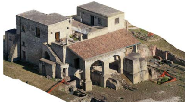
Figure 10: Tempio-Masseria del Gigante, Cuma. 3D model. View from the northwest.
