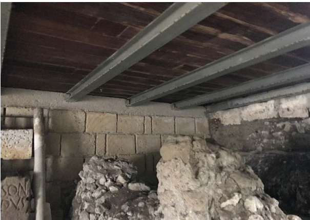
Figure 18: Tempio-Masseria del Gigante, Cuma. The floor in putrelles and wood.
