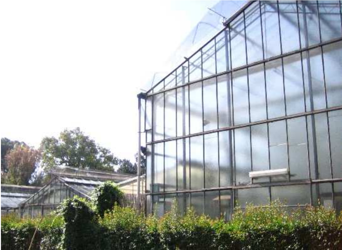
Fig. 14 - View from the outside of the Greenhouse Califano.
